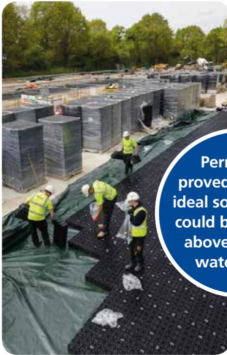
Permavoid proved to be the ideal solution as it could be installed above the high water table.
