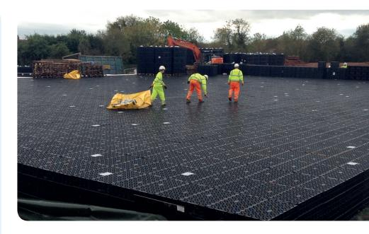
guidelines, meeting the Specification for Highway Works criteria, and capable of attenuating 3,138m³ of stormwater. Installed by Keytec Geomembranes Ltd, the tank was wrapped in geomembrane to ensure the tank remained watertight. This was achieved through Keytec's ability to manufacture large membrane panels, allowing for a quicker installation and reduced on-site welds.
