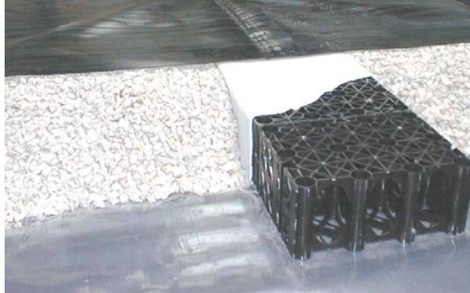
**Figure 1 Permavoid unit within open graded gravel**
