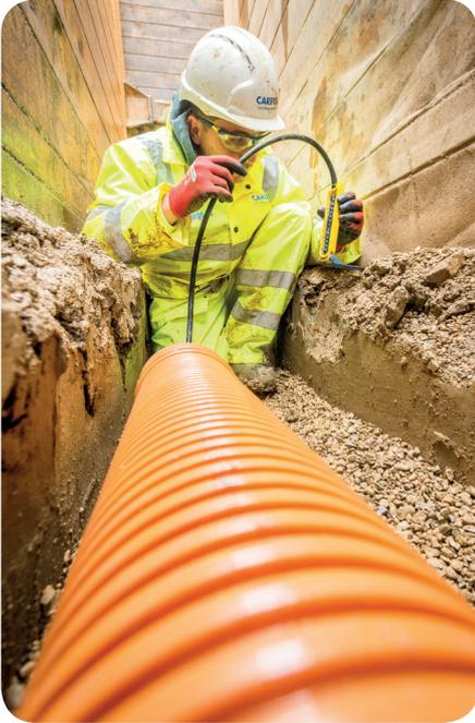
The solution included a system for foul water management using over 2,250m of Polypipe's Polysewer and 330m of Ridgisewer structured wall pipes, along with the necessary associated bends and fittings required to fit the pipe runs.
