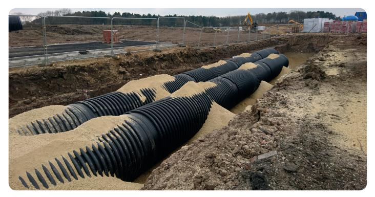
Ridgistorm-XL is designed as a flexible structure to minimise the effects of ground movement, differential settlement and deformation. The pipes are manufactured to meet specific stiffness classes between SN1 and SN8, which was determined following detailed analysis of the site conditions. This flexibility at the manufacturing stage ensured that the delivered pipes will stand the test of time once in position.
