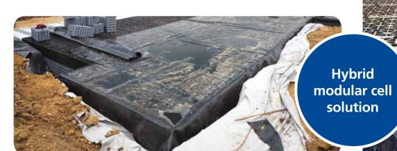
The original project specification included a concrete box culvert. However, following the main contractor's issues with rising material costs and concerns over the performance of the product in times of high-flow water run-off, Polypipe was approached to design a solution capable of storing the required water capacity whilst accommodating difficult site constraints.
