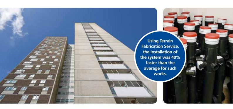
Formerly the tallest building in Southampton, the Millbrook Tower stands at 240 feet. Built over 50 years ago, the building had a cast iron drainage system installed that had started to rust and fail, causing excessive leaking in the 144 flats in the development.
