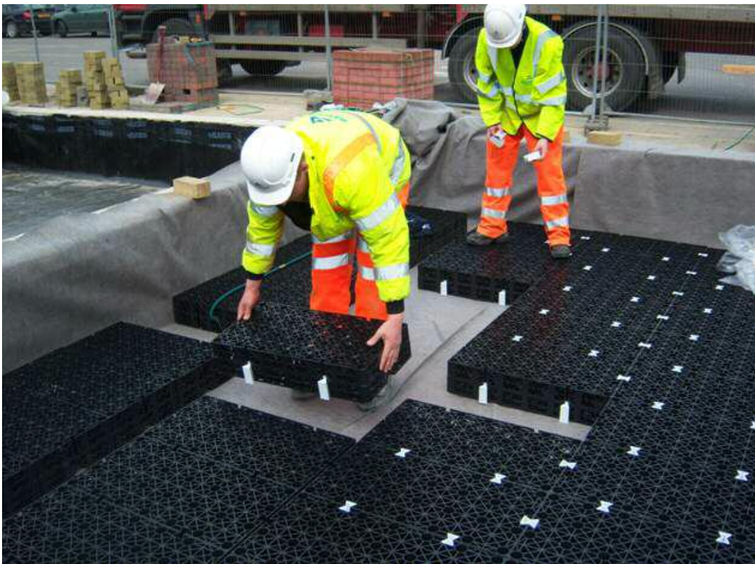
Figure 4.7 Permavoid modular reservoir subbase
