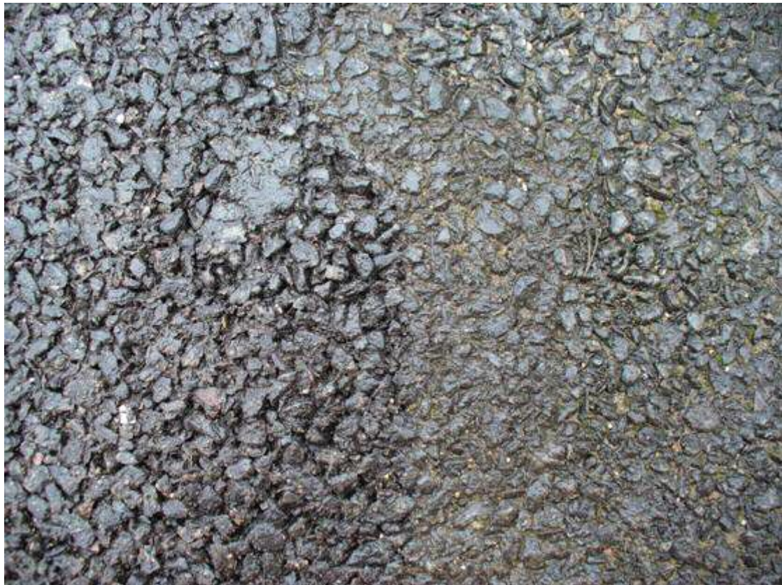
Figure 8.28: Specialist cleaning of porous asphalt
