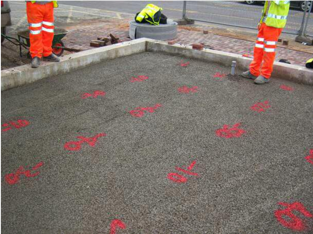
Figure 4.8 Porous concrete base of trial pavements
