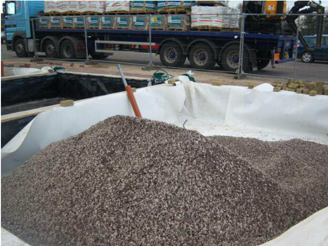
Figure 4.6 Unbound granular reservoir subbase
