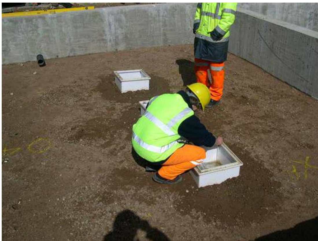
Figure 8.14 Infiltration tests in the imported soil.
