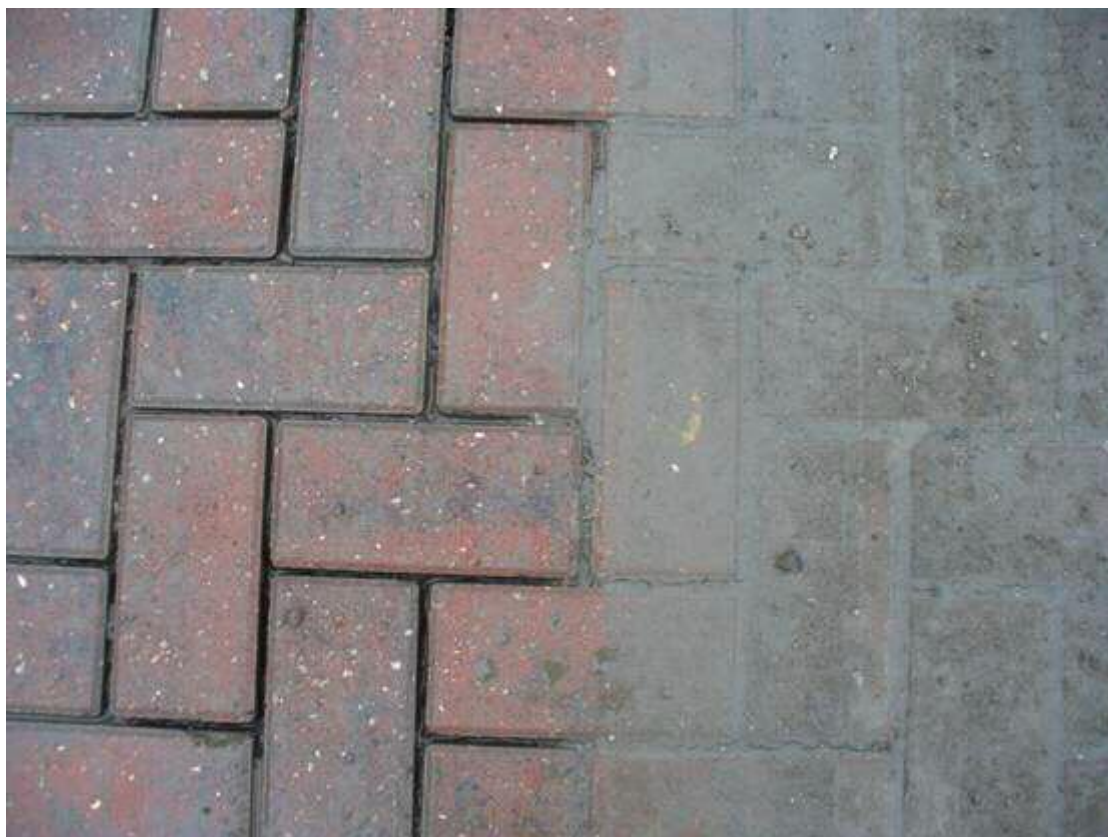
Figure 8.33: Specialist cleaning of block paving
