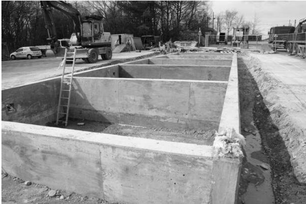
Figure 4.4 Concrete bays constructed to contain the test pavements
