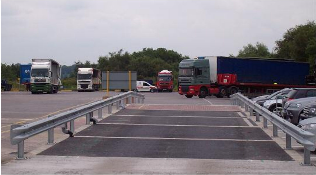
Figure 4.10 Completed pilot-scale trial
