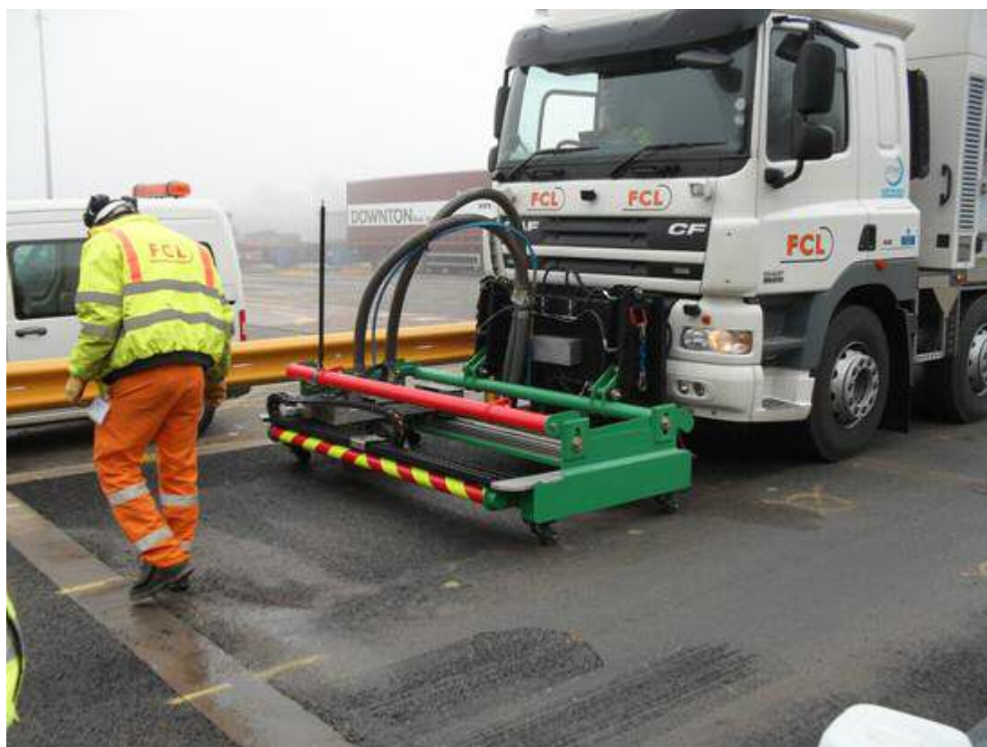
Figure 8.27: Specialist cleaning of trial bays
