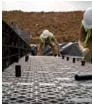
The site, a former private school which has been developed into apartments, consisted of various constraints meaning that the cells needed to be installed on a slope. The solution was a hybrid modular system containing both Polystorm Lite and Polystorm cells which accommodated the differing burial depths resulting in 2,700m<sup>3</sup> of capacity.
