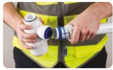
3. When connecting your trap to your waste pipe It's important that the waste can be fully inserted into the outlet of the trap. Once this has been done you can then move the blue finned seal along the waste pipe into the trap.
