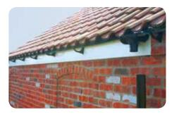
2. Polypipe union brackets and running outlets can be used in place of fascia brackets when the installation allows.
