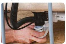
8. To complete the installation, thread the nut onto the outlet. There should be no play in the connection between the outlet and the
