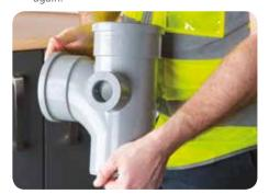
9. After leaving the fitting for 10 minutes, apply solvent cleaner to the inside of the boss connector where the pipe will be inserted. Once the solvent cleaner is dry, apply solvent cement to the inside of the boss connector. It's important that the entire inside surface of the boss connector is covered with solvent cement.
