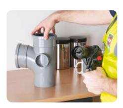
2. Using a drill with a 60mm hole cutter, drill your desired hole.
