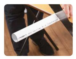
Chamfer the end of the pipe to prevent the ring seal being damaged or misplaced when the pipe is inserted into the socket. Fittings with spigot ends are moulded with a chamfer during manufacture.
