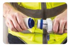
Insert the pipe into the fitting.
