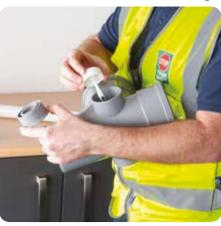
**5.** Also apply solvent cement to the entire outer surface of the boss adaptor.
