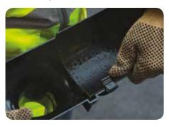
5. It is also important that the gutter is not connected beyond the expansion line which is clearly marked on each fitting.
