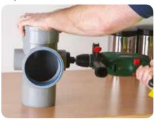
3. Once drilled, remove any loose plastic and de-burr all edges. Apply solvent cleaner to inside surface area of the Boss connection prior to applying solvent cement.
