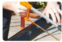
2. After your gutter has been cut we recommend removing any burrs that may be present with a piece of sandpaper. This will stop any loose bits of plastic cutting into the seal.
