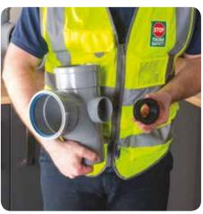
2. Insert the rubber boss adaptor into your boss connection on your soil fitting.
