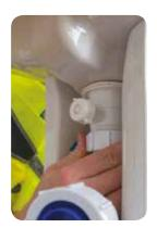
3. If you have installed an adjustable trap as we have in this installation then the trap can be positioned in line with the waste pipe. To do this, loosen the threaded nut below the threaded nut that is
