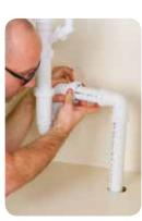
into the trap. Once the seal is in place, the threaded nut can be threaded onto the trap. which will create a compression seal between your waste pipe and trap. After the threaded
