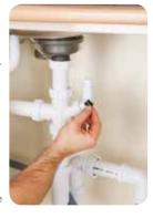
9. Once the cap is removed or the hose end has been cut away, you can connect your hose to the hose connection. Place the appliance hose as far over the hose connection as is possible making sure there are no kinks in the hose once it has rested.
