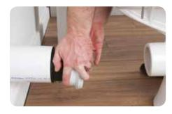
3. Once the pan connector is inserted into the pipe the toilet can be positioned and installed to the pan connector.
