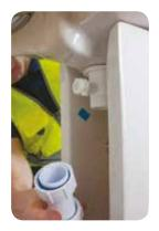
2. To complete the installation, thread the nut onto the outlet. There should be no play in the connection between the outlet and the trap.
