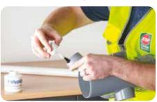
6. Insert the boss adaptor into the boss socket on the soil fitting. Remove any excess solvent cement.
