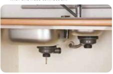
2. Before installing your undersink trap we recommend lining your trap up to all sink connections to make sure you have enough adjustability within the trap and to make sure the outlet of your trap can be connected
