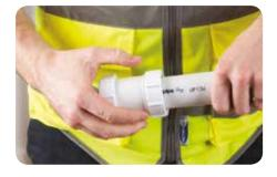
**6.** Screw the threaded nut onto the body of the fitting. Once tight apply an additional ¼ turn.
