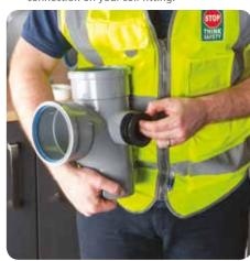
**3.** After inserting the rubber boss adaptor make sure the adaptor is pushed all the way into the boss connection of the soil fitting.
