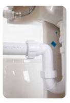
inspection of the connection is required to make sure the connection has been made by pulling on the pipe and fitting. This may not be suitable in certain applications. Once the installation is complete run water through the trap and waste system to confirm the trap has been installed correctly.
