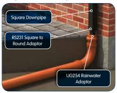
Downpipe discharging into Universal Drain Adaptor
