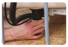
9. Once the installation is complete run water through the trap and waste system to confirm the trap has been installed correctly.
