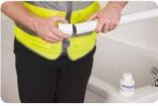
**5.** The spigot should be inserted into the socket immediately, with a slight twisting action.
