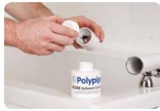
4. Apply a coat of Polypipe solvent cement to both surfaces to be jointed using the brush applicator provided in the lid. The cement should be applied along the length of the spigot and not around its diameter.
