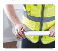
**3.** Lubricate the spigot or ring seal with Polypipe silicone grease or aerosol lubricant.
