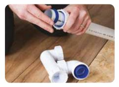
When connecting your bath trap to your waste pipe it's important that the waste can be fully inserted into the outlet of the trap. Once this has been done you can then move the blue finned seal along the waste pipe into the trap.
