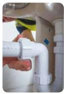
Once the seal is in place, the threaded nut can be threaded onto the trap, which will create a compression seal between your waste pipe and trap. After the threaded nut has been hand tightened a final ¼ turn is required. A final
