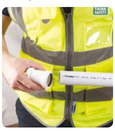
Insert the pipe or fitting into the socket and then withdraw it by approximately 10mm to allow for expansion of the pipework.
