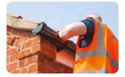
**5.** Connecting to fittings is the same process as in point 4. Prior to connecting your gutter you will need to make sure it does not go beyond the expansion line, which is detailed on each fitting.
