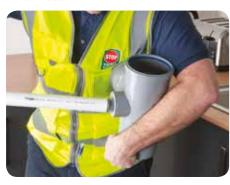
**12.** As with the boss connector it's important to 1/4 turn the pipe once it has been pushed fully into the boss adaptor.
