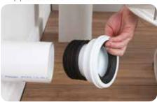
2. Place the finned section of the pan connector into the soil pipe. Depending on the installation it may be more suitable to install the pan connector on the toilet first.
