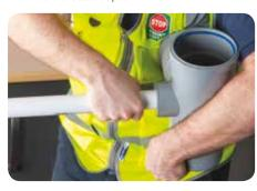
13. Leave your fitting and pipe for 10 minutes before working on them. These parts can be air tested after 24 hours.
