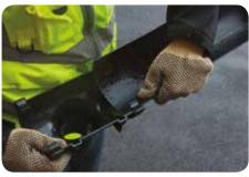
When connecting a piece of gutter to a gutter fitting, it's best to start by placing the gutter under the flexible clip which is facing away from you. Once the gutter is positioned under the flexible clip you can then move the front edge of the gutter under the flexible clip closest to you.
