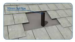
The base plate is dressed to the profile of the lower tiles with the side and upper tiles laid over the top of the base plate. On low pitched roofs, a single welt can be made to the lower edge of the base plate to provide extra strength.
