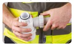
Once the seal is in place, the threaded nut can be threaded onto the trap, which will create a compression seal between your waste pipe and trap. After the threaded nut has been hand tightened a final 1/4 turn is required. A final inspection of the connection is required to make sure the connection has been made by pulling on the pipe and fitting. This may not be suitable in certain applications.
