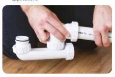
7. When presenting the inlet of your bath trap to the outlet of the bath, the seal must be completely flat to create a 100% seal.
