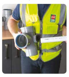
**6.** Once your waste pipe is fully inserted into the rubber boss connector it can be air tested.
