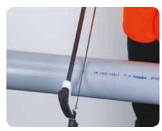
Chamfer the end of the pipe to prevent the ring seal being damaged or misplaced when the pipe is inserted into the socket. Fittings with spigot ends are moulded with a chamfer during manufacture.
