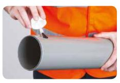
3. Use Polypipe cleaning fluid CF250 to remove any surface grease from the spigot and socket to be jointed.
