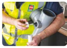
**10.** Also apply solvent cement to your waste pipe ensuring that the entire surface of the waste pipe that will be inserted into the boss adaptor is covered with solvent cement.
