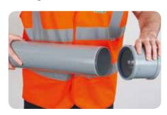
**3.** Lubricate the spigot or ring seal with Polypipe silicone grease or aerosol lubricant.
