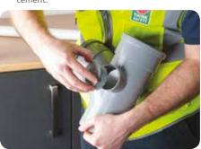
7. Once the boss adaptor is inserted into the boss socket on the soil fitting, ¼ turn the boss adaptor. This process is important as it helps achieve a tighter bond between the boss connector and the soil fitting.
