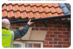
4. Once the back edge of the gutter is in place, the front edge can be clicked into place. It's best to have your gutter in the correct position prior to connecting the front edge as it can be difficult to move the gutter along the run of
