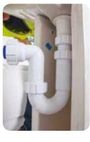
connected to the outlet. Then move your trap either up or down as required, once this is complete re-tighten the threaded nut to re-seal the trap.
