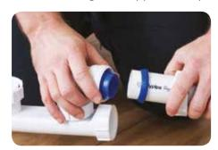
5. Once the seal is in place, the threaded nut can be threaded onto the trap, which will create a compression seal between your waste pipe and trap. After the threaded nut has been hand tightened a final 1/4 turn is required.
