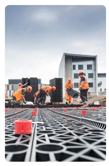
The Permavoid tanks were placed beneath permeable and non-permeable paving, wrapped in geomembrane to make them watertight for attenuation. Permatex, a polypropylene geotextile, was installed between the Permavoid layers to ensure passive water infiltration into the tanks.
