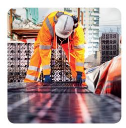
The retrofit SuDS solution will reduce the flooding risk, by protecting properties and basements on the street by intercepting surface water run-off, reducing the flow to the combined sewer system.
