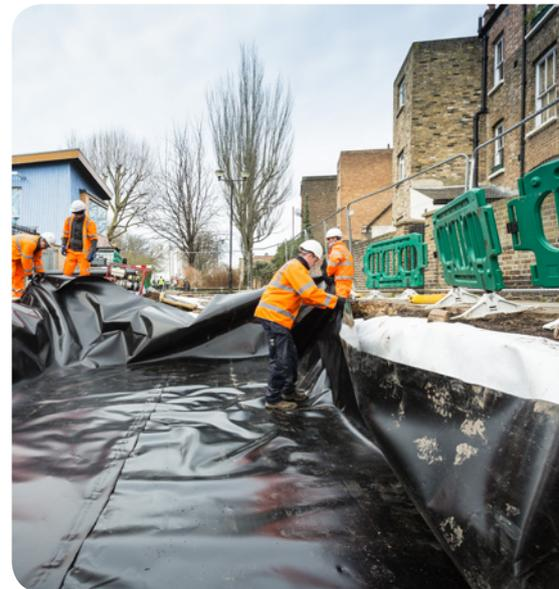
2,345 Permavoid cells have been installed to create four separate storage tanks to sit beneath new rain gardens.
