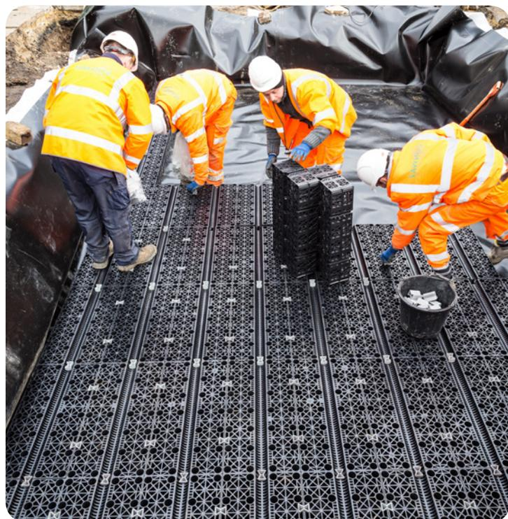
*A total of 430 Permafoam cells were installed to cover a combined area of 108m<sup>2</sup> and will provide water supply for vegetation above. This technique mitigates flood risk during storm events, while sustaining plant growth and providing additional green space in the local urban environment.*
