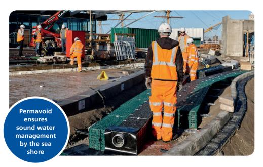
Polypipe supplied a Permavoid engineered shallow water treatment and attenuation solution for Portsmouth City Council's new transport interchange at The Hard.
