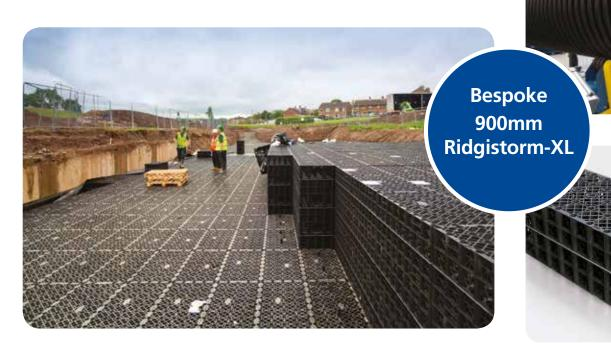
Polypipe delivered its solution for Carrowreagh Storm Sewer Improvement Scheme in Dundonald, near Belfast through an attenuation tank, created from Polypipe's market-leading Polystorm-R and Ridgistorm-XL products. This tank forms an important feature of the £600,000 essential storm water improvement works which are being carried out in response to flooding in a residential area and to meet future Rivers Agency standards.
