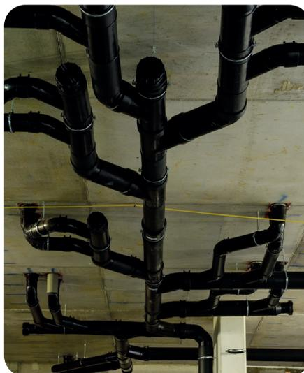
HDPE was specifically used in the in lower levels to avoid the risk of leaks with homogenous welding in the commercial and communal spaces such as the reception area.
