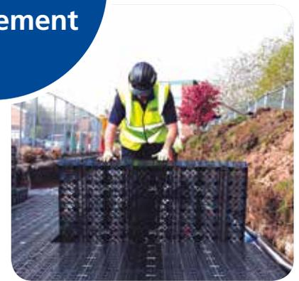
The housing development had previously flooded during heavy rainfall due to interaction between surface water sewers and the water level in the nearby Ouseburn River. To help prevent future flooding, Polypipe's Permavoid system was installed under a recreational area between a road and the river.
