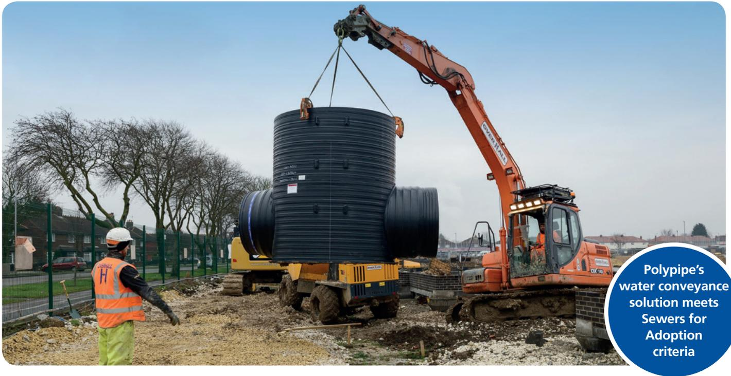
Polypipe delivered a system that demonstrates how large diameter pipes can meet strict Sewers for Adoption guidelines, while managing the traffic load from the road infrastructure.
