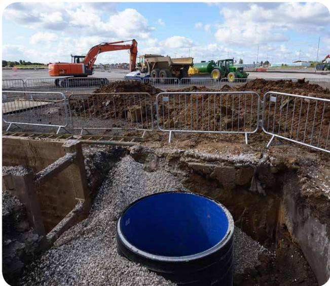
“ Ridgistorm-XL was supplied in a variety of stiffness classes in order to provide a robust solution to compensate for the varying ground conditions found on-site, including soft clay soils, as well as loading above from vehicles. ”
