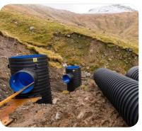
In a demonstration of its versatility, robustness and light weight nature versus traditional materials, Polypipe's Ridgistorm-XL large diameter piping system has been airlifted up the mountainside of the Arrochar Alps to Loch Sloy as part of a rather unusual power sector project.
