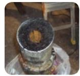
These are actual cast iron soil stacks removed from a high rise Local Authority building where ongoing system breakdown has caused these kinds of sanitation issues, such as leaking and blocked pipes.
