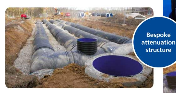
Developer Pentland Homes required a drainage solution which controlled water discharge at a rate of 4 litres per second into an Environment Agency managed watercourse.
