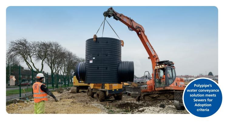
Polypipe delivered a system that demonstrates how large diameter pipes can meet strict Sewers for Adoption guidelines, while managing the traffic load from the road infrastructure.
