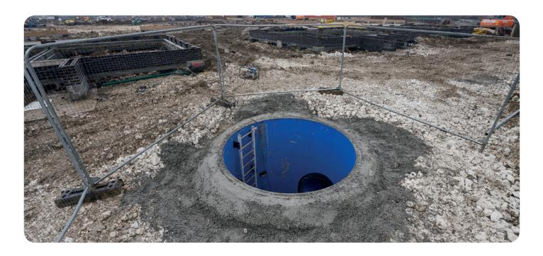
"Polypipe provided a value engineered solution using Ridgistorm-XL tanks, with pipes manufactured to the perfect stiffness classification to meet our needs, together with convenient pre-fabricated pipework and manholes. "This solution met the requirements of Yorkshire Water and Hull County Council, while also providing a robust and efficient system ideally suited to the development's challenging conditions." **Trevor Smallman, Project** Manager at Keepmoat Regeneration.
