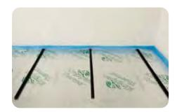
It is not necessary to overlap the clip rails. They can be clipped together end to end to form longer lengths.
