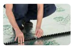
Continue to fit the clip rail across the room at 1m intervals making sure that sufficient space is left around the perimeters of the room (approx. 800mm) to accommodate any pipe returns or connection lengths back to the manifold. Care should also be taken to ensure that the clipping alignment is maintained.
