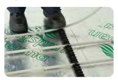
If necessary use an additional clip or pipe staple (PB02930) to firmly secure the 180° return bends.
