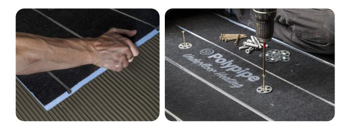
Depending on the type of substrate, the Polypipe Overlay<sup>™</sup> Plus or Polypipe Overlay<sup>™</sup> Plus Acoustic can be fixed with screws and washers or a continuous bed of flexible tile adhesive. It is essential that the floor onto which the panels will be fixed are flat and exhibit no movement. An uneven floor must first be made flat using a levelling compound.
