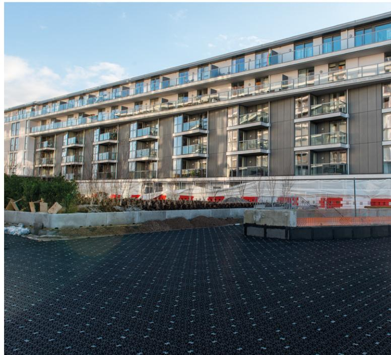
27,600 Permavoid units were used in total, and ideal for the shallow environment available to install the system. And because they are lighter in weight than traditional materials, and have high void ratio, they negated the need for heavy concrete basement tanks. But despite its light-in-weight properties, Permavoid is exceptionally strong – allowing amenity for car parking and maintenance vehicle traffic above, whilst clever water management continues below.
