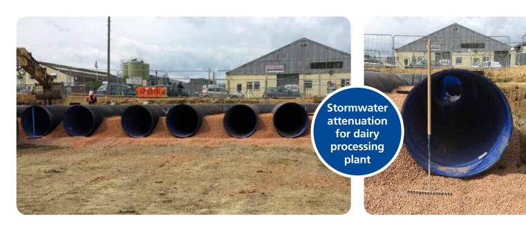
As part of a large-scale renovation to increase yard space, Cotteswold Dairy has seen Polypipe's thermoplastic Ridgistorm-XL solution utilised to capture and attenuate excess surface water and potential milk leakages. Working closely alongside Vitruvius, the project's Construction and Cost Management team and main contractor Smith's of Gloucester, Polypipe fabricated over 250 metres of Ridgistorm-XL, incorporating a RIDGISTORMCheck Vortex Flow Control Chamber, to sit beneath the lorry park.
