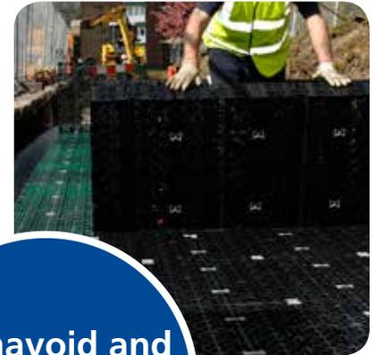
Permavoid and Permafilter Geotextile
