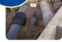
Polypipe supplied two of its Ridgistorm-XL pipes, designed to suit the site-specific requirements of the project to consolidate three existing CSO chambers into one. The large diameter pipes were designed to an exact specification of 1800mm and 1200mm. Through analysing the site conditions and parameters, Polypipe's technical design team were also able to identify a lower stiffness classification of SN1, resulting in a cost effective solution that was neither over nor under specified.
