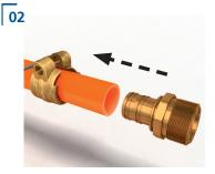
Push the fitting insert completely into the medium pipe until it reaches the collar of the fitting.
