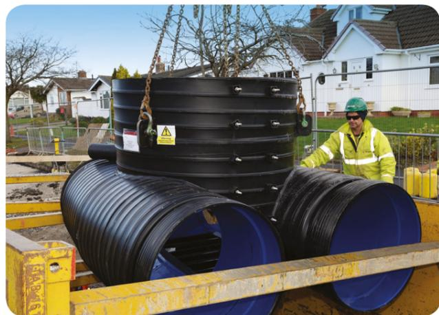
As well as providing Ridgistorm-XL pipes in 900mm diameters, we were able to pre-fabricate structural components to create a number of 1500mm RIDGISTORMAccess Multiple Pipe Manholes, allowing dual carrier pipes to run parallel to one another. The manhole access was positioned centrally to allow for a single point of access into both pipelines.
