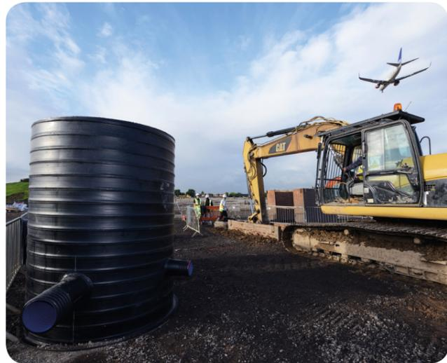
The drainage system covered an area of over 65 acres, using surface water drainage pipes from 150mm Ridgidrain to 1200mm Ridgistorm-XL large diameter pipe and over 100 component chambers. The drainage system allows captured surface water to be carried through a number of drainage runs and pre-fabricated chambers before entering an existing water course.
