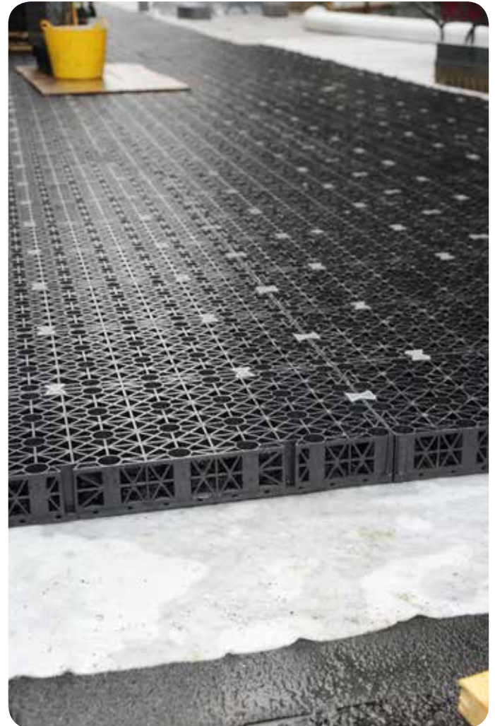
Typical Permavoid Sub-Base Replacement System v Traditional Aggregate Sub-Base
