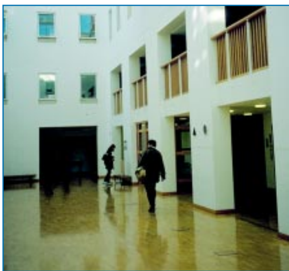
Above: An example of timber flooring used to cover an underfloor heating and cooling installation. The nature of expected pedestrian traffic will directly influence the choice of screed. The heavier the traffic, the stronger the screed.
