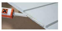
When gluing the ends, ensure there is no residual glue in the pipe grooves and use short lengths of pipe to help with panel alignment.
