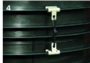
4 The Risers are now secure
