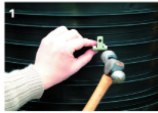
1 Attaching fixing kit clip (FRK503)
