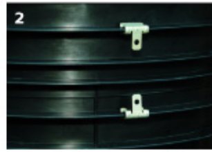
2 Clips should align for fixing
