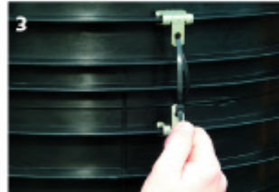
3 Pass jointing tie through clips and tighten
