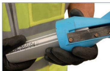
Remove any debris left after cutting and de-burr using a de-burring tool or reaming tool.
