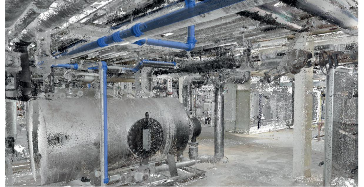
3D scan demonstrating how Polypipe can add value to your retro fit projects by scanning your building and overlaying with the exact MecFlow pipes and fittings you would need to complete your job.
