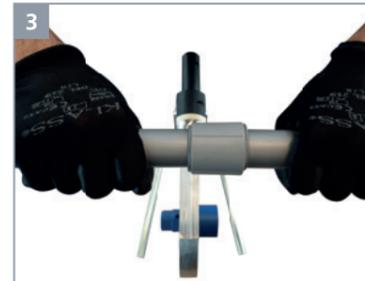
3. Once the heating time is reached, remove the pipe and fitting from the hot plate, and immediately push them together, without twisting, to the insertion depth marked on the pipe. This must be completed within the joint time listed in table 6.04. Continue to hold the pipe and fitting together for the duration of the cooling time specified in table 6.04.
