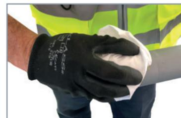
Dirt and oil can be removed from the pipe's surface using an isopropyl alcohol-based cleaner (91% by volume or greater).
