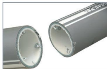
Once a cut is made, check the ends of the pipe for damage, both internally and externally. If any damage is identified, mark and remove the damaged area, cutting a few millimetres beyond the damage.
